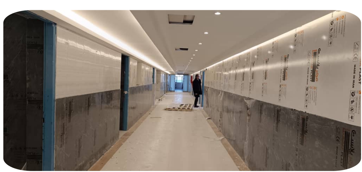
Zahedan Cleft Center of Excellence under construction.
